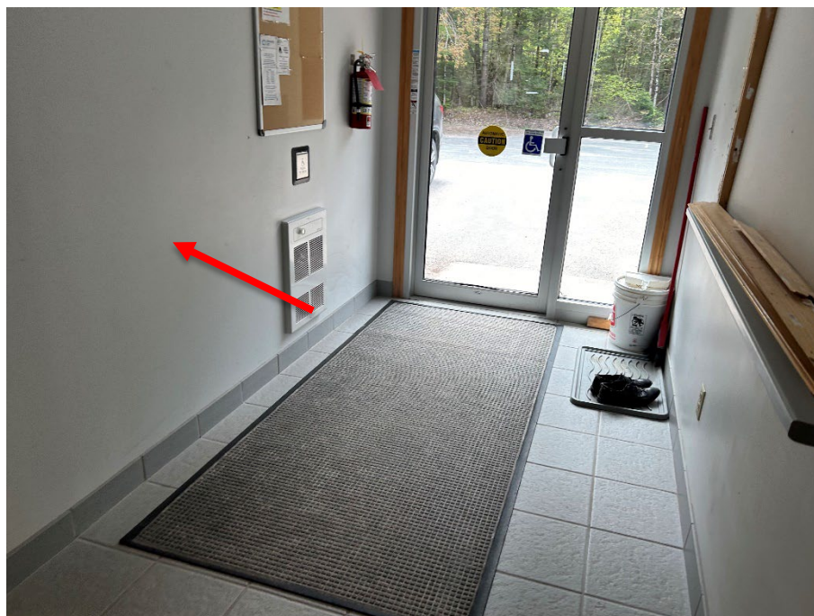
Photo 1 – Non-asbestos drywall joint compound.
